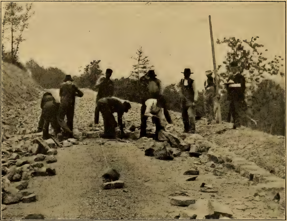
Laying a Telford foundation for a hillside highway.
